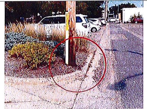
Photo 6 - Curbing within the TE area. (Curbing is in Poor Condition)
